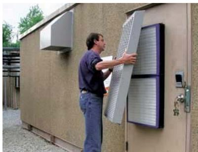
Figure 1. Door-mounted Intake Filters (right) and Exhaust Plenum (left).
